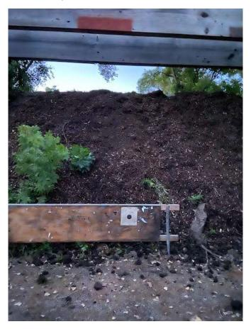
In the fall of 2020, we were able to get an excellent price on fill. We received 52 truckloads of fill and used it to build the height of our berm. The berm is now twice the height that it was. While we haven't measured it yet, it should be close the height recommended by the NRA for a berm. We hope to get as good a deal this spring and build it a bit higher.
